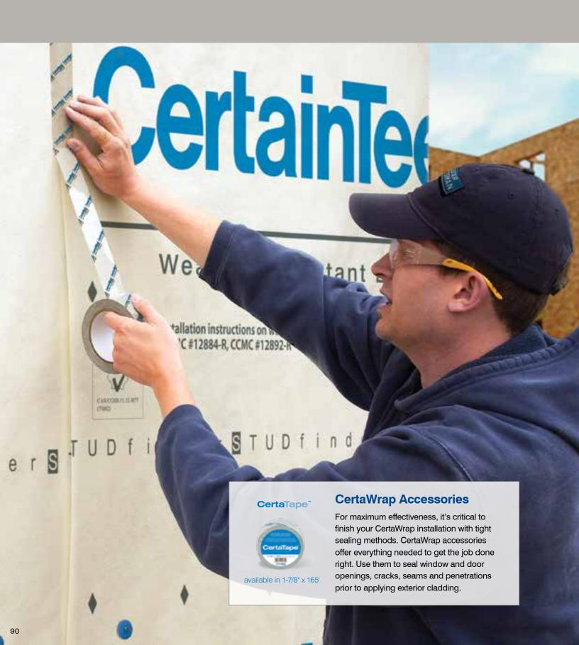
CertaWrap Weather Resistant Barriers, in premium or standard grade, provide an added layer of protection against air and moisture damage. It's part of the complete CertaWall Weather Deterrence System™.
